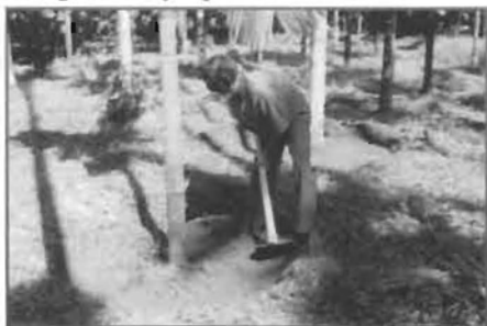
Raking the basin
